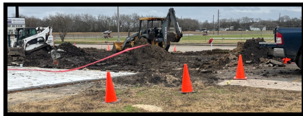
West end driveway
