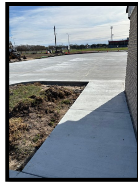
Sidewalk and side parking lot
